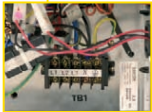
Outdoor unit power supply terminal block
